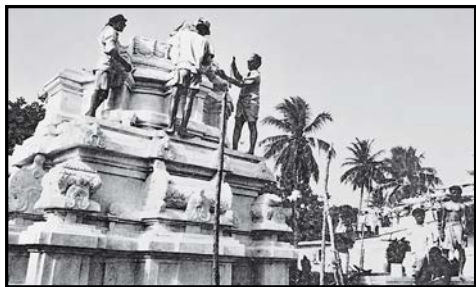
Renovation at Jeevaratna Vinayakar Temple
