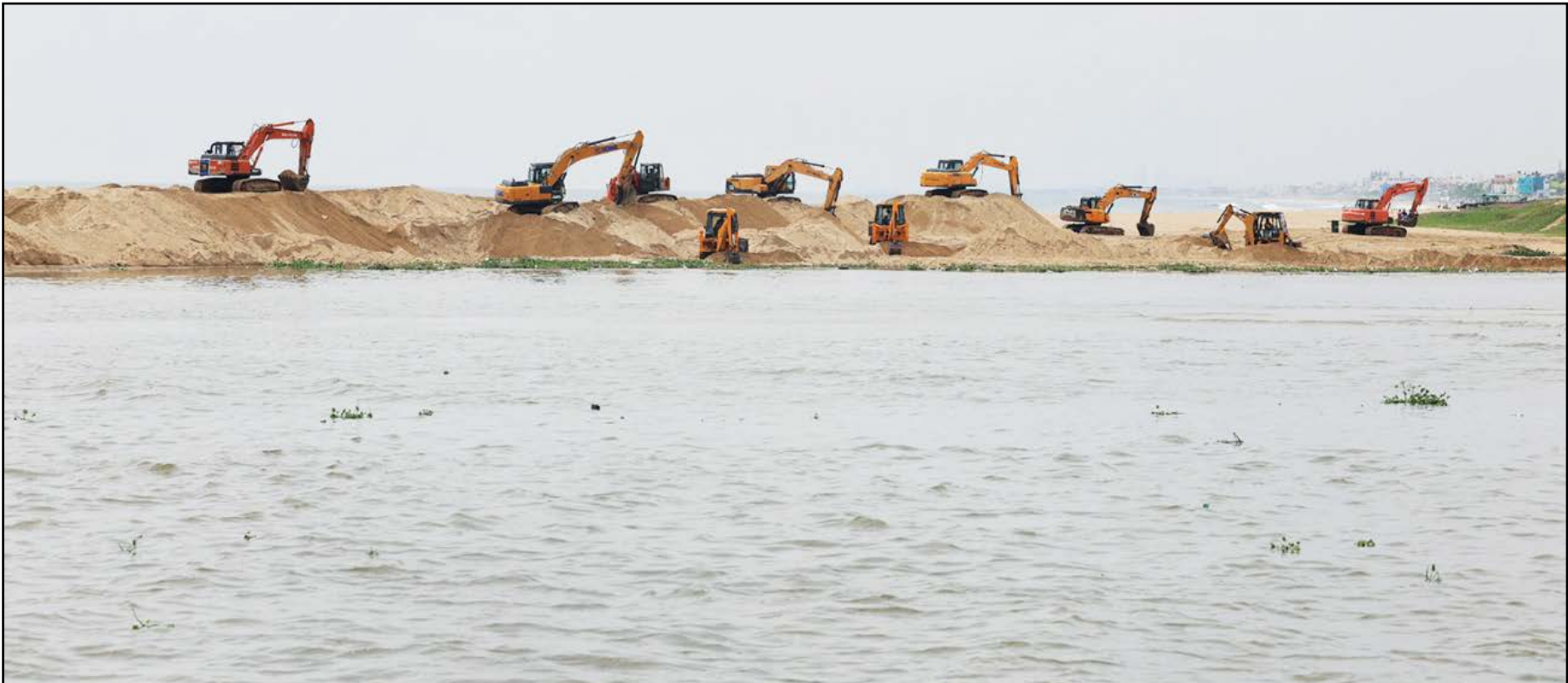
JCBs remove silt which clogs the mouth of the Adyar river at points off Srinivasapuram / Pattinapak-kam on the northside of the river and Besant Nagar’s Urur kuppam on the southside. The mounds of silt affect the free flow of water in the river into the sea when the volumes grow at monsoon time.
