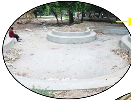
● INTERACTIVE SPACE - the only progress evident is the mortar circular structure around the giant peepul tree. The metal beams to support the roof are still being fixed.
