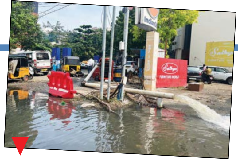
Stagnating water that sank the P S Sivaswami Salai zone, Mylapore was pumped into the drain off R. H. Road to be led into the Canal. Stop-gap solution for the worst-hit area of Mylapore executed three days after the havoc.
