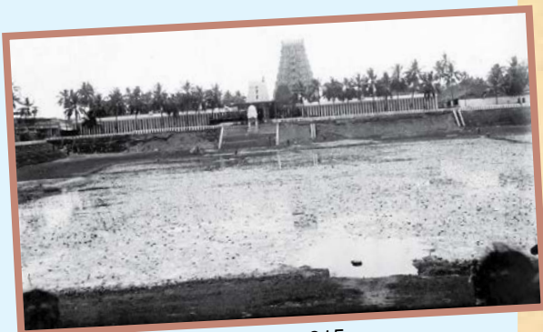
● Steps under construction 1915
