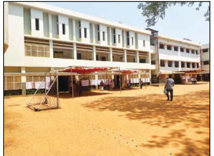
A deserted Vidya Mandir school campus at 1 p.m. Five booths here.
